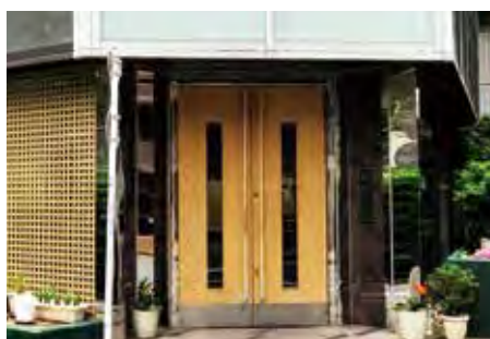
Entrance of Building No. 1
