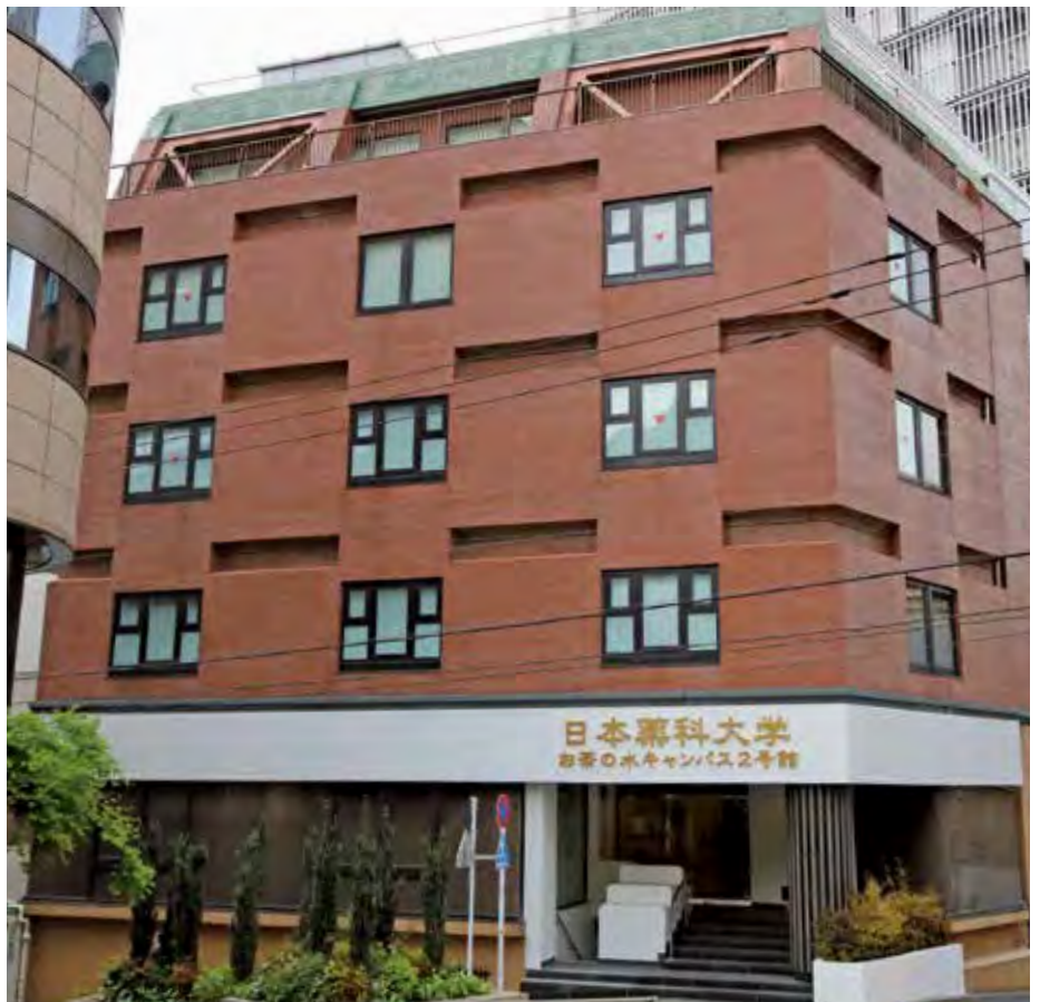
Exterior appearance of Building No.2
