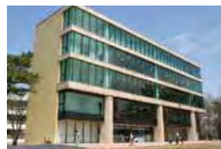
Cafeteria and Welfare Building
