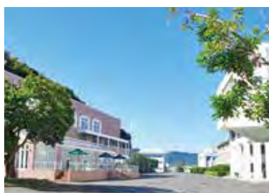
Daiichi Institute of Technology, Kagoshima Campus
